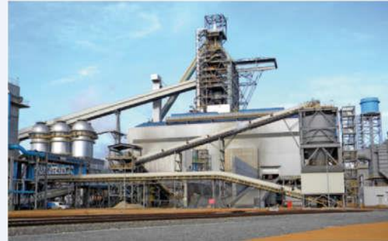
Cowper recuperators: Steel
