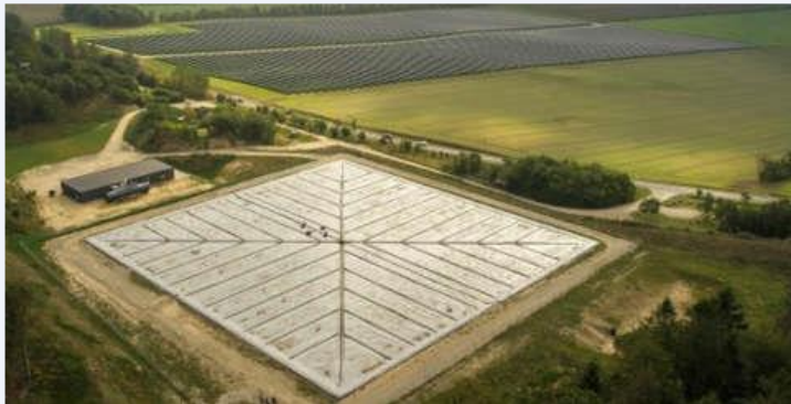
DK; pit storage; solar
